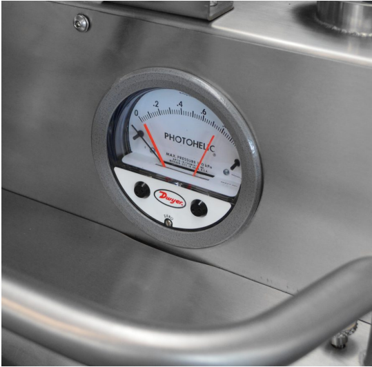
Photohelic filter indicator sensor for Delfin PHARMA 40.40
